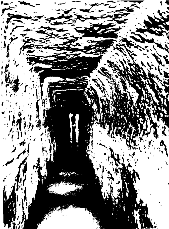
3. The Siloam Tunnel (cf. 2 Kings 20:20).
